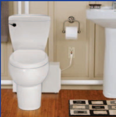
3 System and Plumbing Exposed
