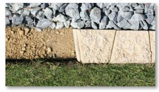
Step 1 Lay out the line or curve you would like your edging system to follow. With a spade or flat shovel, dig a shallow trench to approximately 3" deep by 6" wide to receive the edging unit. Prior to placing the units, provide a layer of land-scape fabric in the trench, below and up the sides of the Keystone Insignia<sup>TM</sup> Edger.
