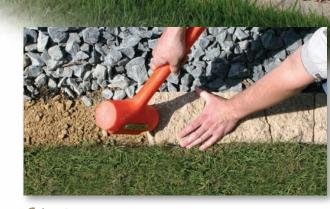
Adjust unit alignment by hand or by using a rubber mallet to tap the units in place. Finalize your installation by placing landscape rock, mulch, sod, or other similar materials to achieve your final design appearance.
