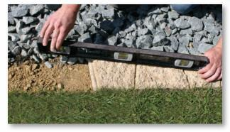
Step 2 Place units in the trench, over the landscape fabric, in either a straight line or a curved alignment. Interlock the overlap edge detail of the A & B units in an alternating manner to connect the system to its final geometry.
