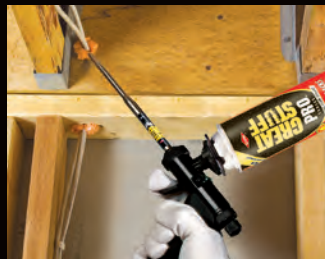
Electrical wire penetration
