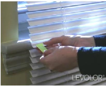
Step 3: Pry all the plugs from the underside of the bottom rail
