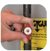
With the gas control valve switch Off, turn the gas supply valve ON. Brush soap solution on all gas line connections and look for bubbles. Use plenty of soap solution. Gas is under low pressure, and it may take some time for bubbles to appear. If you see any bubbles, turn Off the supply gas valve and (most don't need pipe joint correct the leak. Then turn On the supply gas valve and retest. Then turn the gas supply valve back ON and retest. Do NOT check with an open flame.
