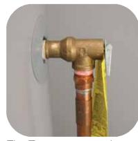
The Temperature and Pressure Relief Valve (T&P) is an important safety device. It opens to relieve temperature or pressure if the water temperature or pressure is inches between the end too high. Use the new T&P that came with your new water heater. Don't reuse the old T&P valve.
