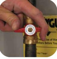
Turn off the gas supply to the water heater at the manual shut off valve. Turn gas control knob to the OFF position. Disconnect the gas line at the union (you'll need two wrenches for that). Remove the gas pipe from the old water neater—you may be able to reuse it. Save the union, too.
