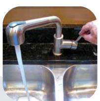
Open a hot water faucet and let the "hot" water run full for at least three minutes to ensure the tank is completely full of water. Check all connections for water leaks. Almost all leaks are at the connection points, not a tank leak.
