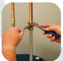
Install the hot and cold water lines. If using quick connect fittings, pipe compound or Teflon® tape is not required. If using flexible or solid connections, the threaded fittings require pipe compound approved for potable water or Teflon® tape on the threaded fittings. Turn the cold water supply back on and check for leaks. Do not solder pipes while they are connected to the water heater, use threaded adapters.
