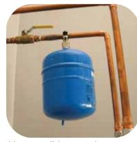
Almost all homes have check valves in the plumbing system and homes now need a thermal expansion tank installed near the water heater. The expansion tank is attached to the cold water inlet line. To operate properly, the expansion tank must be pressurized with air. Refer to the expansion tank's instructions for details.
