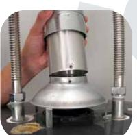
Be certain that the vent has cooled before handling. Disconnect the vent pipe from the draft must have free access to adequate combustion air and must be properly vented. The Installation Instructions explain these requirements, and they must be followed for safe operation.
