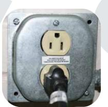
This residential gas water heater requires a 120VAC, 60 Hz electrical supply. A 10-foot cord with 3-pronged plug is supplied (no extension cords are permitted) and the outlet must be properly grounded. Follow local codes. See Installation Instructions for details.
