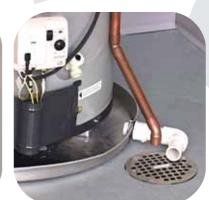
The Temperature and Pressure Relief Valve (T&P) discharge pipe should be terminated near a floor drain with an air gap of no more than 6 of the discharge pipe and the drain. Some localities require terminating the T&P discharge pipe outside. In cold climates, we recommend using a floor drain. In all cases, follow local codes. Read the Instruction Manual for important details. Warning: Do not plug or cap the T&P discharge pipe.
