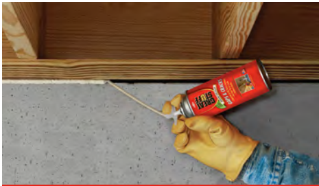
Rim joist/sill plate
