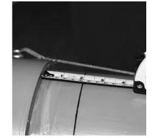
To ensure joint integrity, once insertion is complete, the pulling tool can be used to hold the joint in place during set time and also to ensure that the pipe does not back out.
