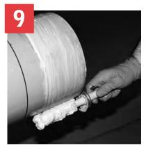
Apply a medium layer of cement to the fitting socket aggressively working it into the surface. On bell end pipe do not coat beyond the socket depth.
