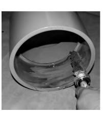
• **NOTICE:** Pipe diameters 6" and larger must be installed using IPS P-70 or Oatey Industrial Grade primers.
