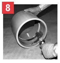
Apply primer to the pipe surface to a point ½" beyond the hub depth. Aggressively work the primer into the surface.
