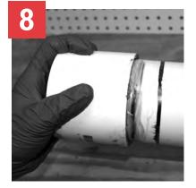
• Insert pipe into the fitting hub
