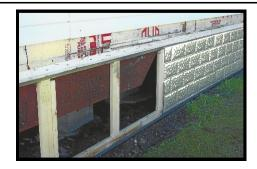
Framework consists of 2" X 4" boards placed 5' apart or 30" on center. Pipe grips secure rebar sections that have been anchored into the ground.
