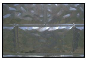
Using the spaces between the block pattern as a guide, you may fasten skirting to framework with either a hammer and galvanized roofing nails (with rubber washers) or with stainless steel screws as seen in the
