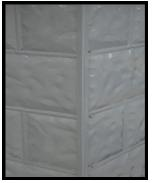
Corners can be made by bending skirting around or into the corner or can be trimmed and J-channel used along the top, bottom and end edges of
