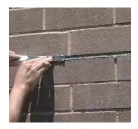
Using a joint tool, insert it into the joint and slowly drag across the joint. Apply additional mortar, if needed, to ensure the joint is completely filled.
