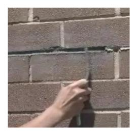
Turn the tool sideways and scrape off any excess mortar.
