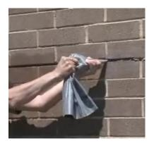
Insert the tip of the grout bag into the joint and squeeze.
