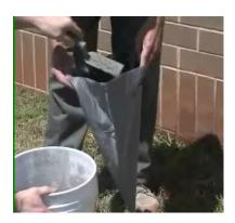
Fill grout bag with mortar. Using a grout bag allows for increased accuracy and reduced mess versus using a trowel.
