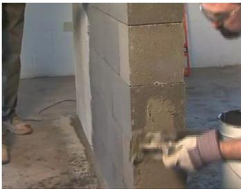
To achieve the structural potential of Surface Bonding Cement for mortarless block wall installations, proper applications should be 1/4" to 5/16" of material around all sides and ends of the area and in uniform thicknesses throughout.
