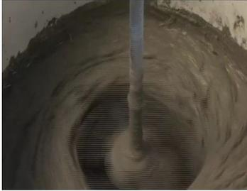
Mix the Surface Bonding Cement according to the mixing instructions on the back of the bag.
