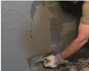
Now that the surface of the block has been dampened, start at the base of the wall and trowel upwards with the Surface Bonding Cement in even coats with the minimum thickness being no less than an 1/8" thick.
