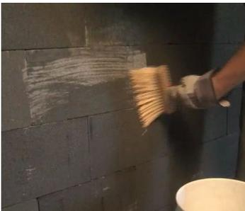
Before applying the Surface Bonding Cement, dampen the surface of the block. This will aid in the adhesion of the material to the block and will also eliminate the otherwise dry block from pulling the moisture out of your Surface Bonding Cement mix.
