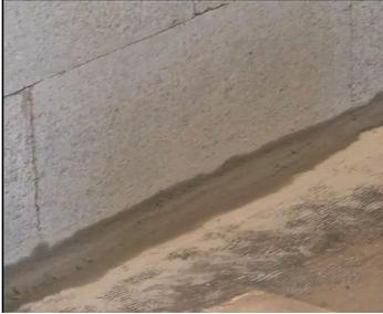
Prepare a mortar bed to secure the first layer of block. Be sure the mortar bed and first course of blocks are level.
