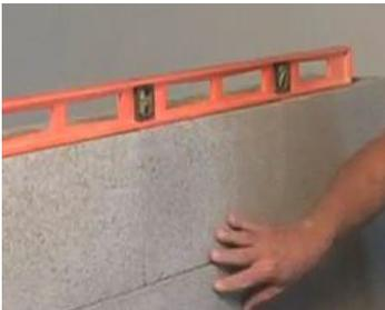
Through out this block stacking phase and at the completion, check that the wall has remained level.
