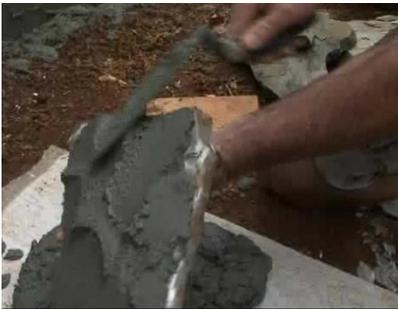
Apply mortar to the back of the stone and begin setting stones at the lowest point on the wall and work up. It is best to begin at the corner.
