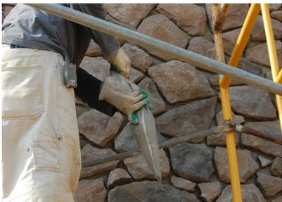
Add mortar to the joints between the stones using a grout bag.
