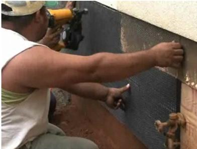
Install a moisture barrier prior to installing stone veneer.
