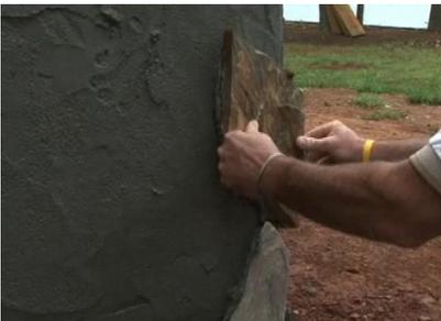
Press the stone firmly in place using a twisting motion and hold in place just long enough to be sure it does not slide.
