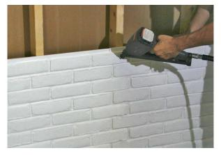
Continue with the rest of the panels of the first row. If the faux brick panels terminate against another wall, simply cut the panel to size. The exposed edges will be hidden by the next wall. It is always better to mark your dimensions in the back of the panels to make cuts. You may also caulk any joint between panels and touch them up with paint. We recommend starting the next and all odd rows with half panel in order to stagger the vertical seam and creating a better flow.
