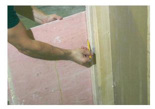
It is now time to install the mitered pieces. Apply the construction adhesive on the inside of one of the edges, or both. Secure the two pieces over the substrate with a finish nailer or screws
