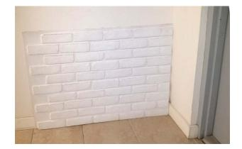
We strongly suggest securing the panels with construction adhesive (Liquid Nails, PL Premium etc.) as well as fasteners such as screws or nail. The brick panels may be installed directly over drywall, plywood or framing. In cases of bare framing apply the adhesive on the framing itself. When installing on a flat surface the adhesive may be applied on the back of the panels:
