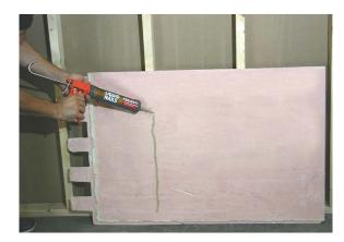
Secure the panel on the substrate using screws or finish nails (using nails will help to conceal the heads). It is important to apply plenty of adhesive on the flat overlapping areas, where panels overlap, to have strong bond between panels.
