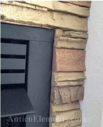
2- Some customers sand and file the cut edges and shape them to look like the ends of a real stone. They apply some textured caulk and paint the caulking with our Touch-Up kits.
