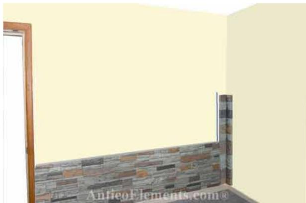
Continue with the rest of the panels of the first row. Trim the right end of the last panel (for the Laguna it would be the left end) to fit against the wall corner. It is always better to mark your dimensions in the back of the panels.
