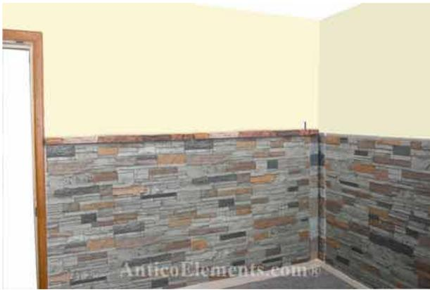
Install the [Top Sills](#) in the correct direction making sure to locate the unfinished edge and placing it against the wall. The bottom front edge should be the finished one. If the sill isn't touching the wall it should be turned around. To create a better seam between two sill pieces that merge at an angle, the sills should be mitered where they meet at the corners.
