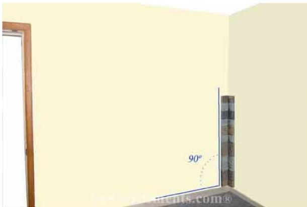
It is always a good idea to temporarily lay out the panels around the project to plan which / how panels will be cut and which will not.
