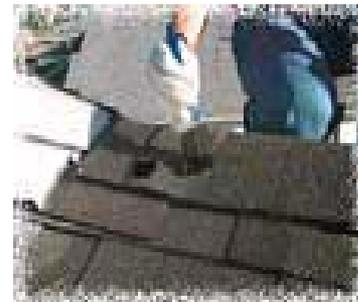
When completing a cap of shingles, the last cap will have exposed nail heads which need to be covered with **Black Jack Roll Roofing Adhesive**.
