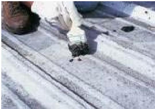
Corrugated roofing sheets are often nailed into place leaving a path for water to leak through.
