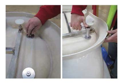
6. Use the levelers on the pedestal to make any needed height adjustments.
