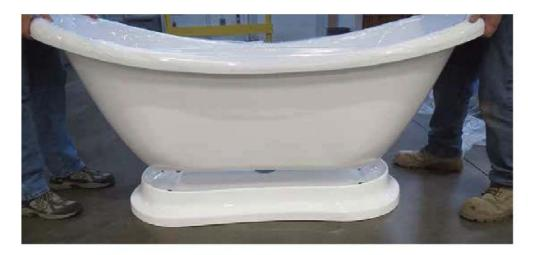
5. Once dry, turn the tub and over and re-attach the hardware. Be careful not to over-tighten the bolts.
