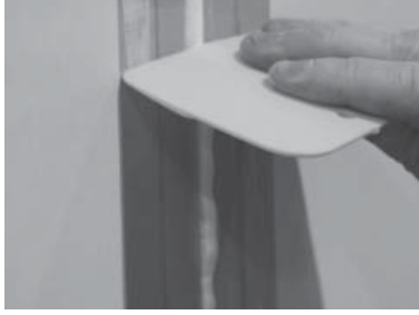
FIGURE 18: REMOVING EXCESS SEALANT
