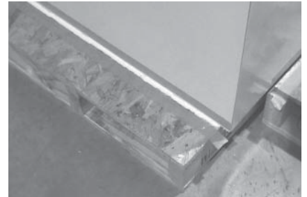
FIGURE 22: HORIZONTAL SEAM FILLED COMPLETELY WITH SEALANT
