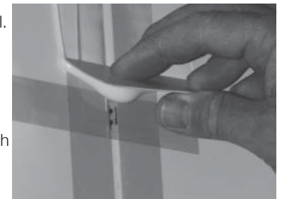
FIGURE 17: APPLYING THE PAINTER TAPE HORIZONTAL IN 3' SECTIONS
