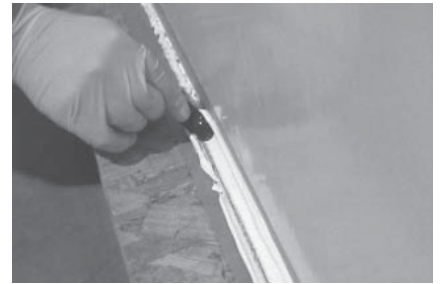
FIGURE 23: HORIZONTAL FINISH WITH ROUNDED CORNER
