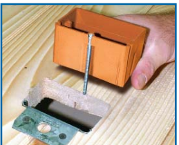
Install clip over subfloor.
