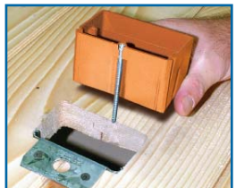
Install clip over subfloor.
