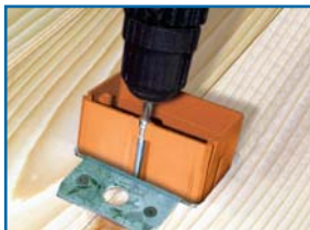
Screw in to adjust to height of flooring or carpet.
