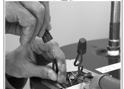
Connecting the electrical wires.
