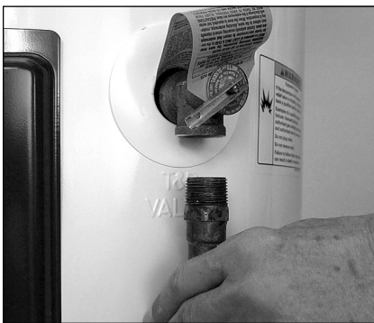
Removing the T&P Relief Valve discharge pipe.
