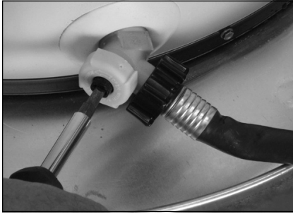
Draining the old water heater.
