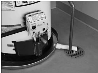
Figure 23 - Metal drain pan piped to drain.
