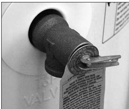
Figure 25 - Temperature and Pressure Relief Valve
