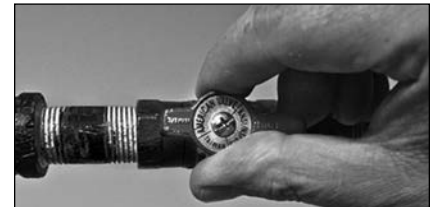
Figure 58 - Gas valve in “on” position.
