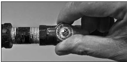
Figure 32 - Gas valve in "on" position
