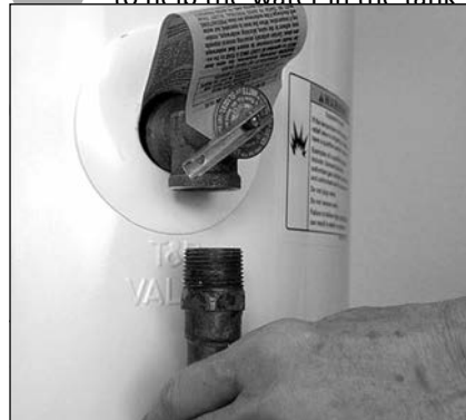
Figure 21 - Removing the T&P Relief Valve discharge pipe.
