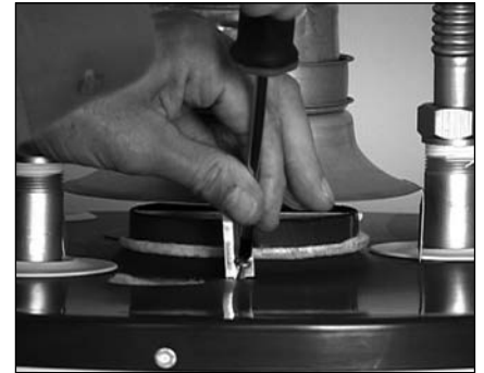
Figure 30 - Install the new draft hood and secure with screws.
