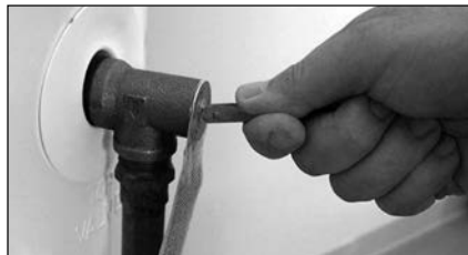
Figure 45 - T&P Relief Valve.
