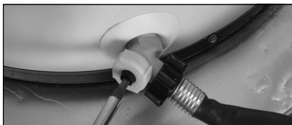
Figure 42 - Draining the water heater.
