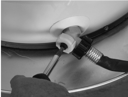
Figure 10 - Draining the old water heater.
