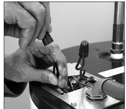
Figure 19 - Connecting the electrical wires.
