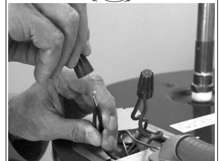
Connecting the electrical wires.
