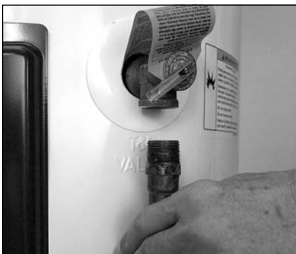
Removing the T&P Relief Valve discharge pipe.
