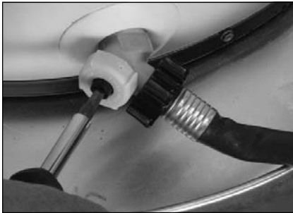
Draining the old water heater.
