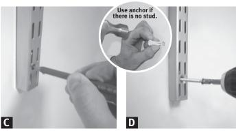
**Secure** Mark bottom hole of each upright. Drill 1/8" pilot hole into stud. (Use wall anchor and 3/8" bit if there is no stud.) **Fasten at bottom** Fasten screws into studs or wall anchors. Screws are needed only in bottom holes of uprights.
