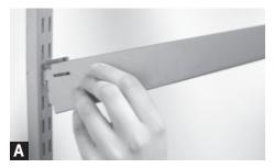
Insert brackets Insert brackets into uprights at desired locations. Note: Install brackets and shelving at the top first and work down. Brackets will not fit into upper two slots of each upright.
