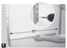
**Use 22" rail cover for spacing** Hang another 47.5" upright on the rail and use one of the 22" rail covers to space over 22". Drill 1/8" pilot hole and fasten screws in bottom hole. (Use wall anchor and 3/8" bit if there is no stud.) Place 22" rail cover over rail between uprights. Repeat step **F** for additional upright (if space allows).
