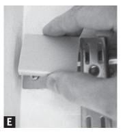
Attach 6" rail cover Clip 6" rail cover over hang rail so uprights stay in place.
