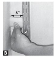
**Position at 6"** Position both outside uprights 6" from the right and left corners by using the 6" rail cover for spacing.
