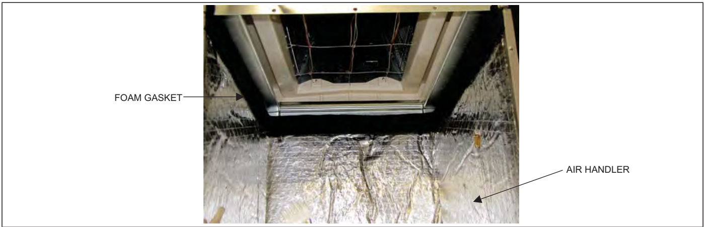
FIGURE 4: Gasket Location
