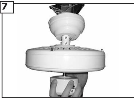
7 Hang assembled fan from the mounting bracket installed in ceiling in previous step. Make sure the fan is hanging straight. Rotate fan until the tab on the Mounting bracket engages the slot on the Downrod Ball. This must be done to prevent the fan body from rotating when the blades are in motion.
