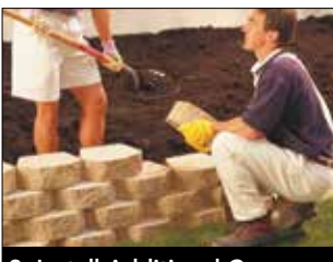
3. Install Additional Courses
