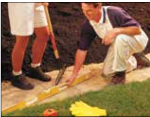
1. Prepare Wall Location
