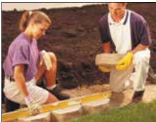
2. Place & Compact Backfill
