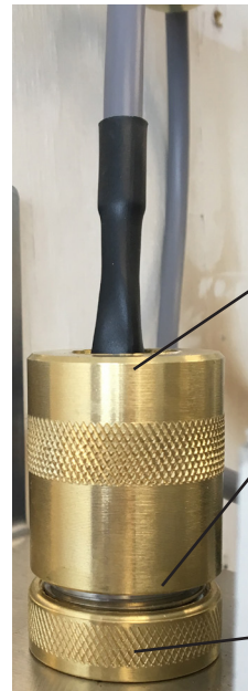
2) Quartz Sleeve inserted into UV Chamber
