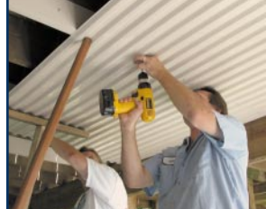
Fije paneles DeckDrain
