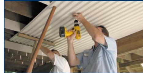
Attach Drain Panels
