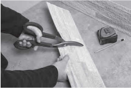
Cutting a straight cut with a snip
