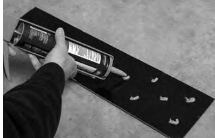
Method 2 - Using high-quality polyurethane construction adhesive
