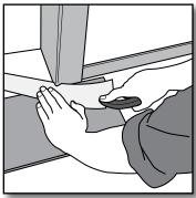
[2] Undercut doorjambs for a professional fit. Doorways less than 6' wide require T-Molding.
