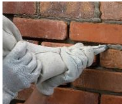
Installing Thin Brick and filling in joints
