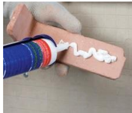
Installing Thin Brick and filling in joints
