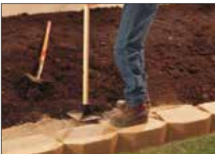
2. Place & Compact Backfill
