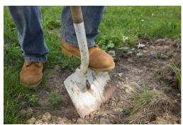
Dig a trench approximately 4"(101.6mm) deep by 12"(304.8mm) wide to your desired length and shape, (straight and/or curves) being sure to remove large rocks, roots, organic material, etc.. If the soils contain organic loam, dig an additional 4"(101.6mm) deeper and add a compacted gravel or sand leveling pad 4" (101.6mm) thick.
