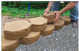
Begin placing the second course of block at straight wall areas being sure to center each unit over the joints of the blocks below in a "running bond" or 1 over 2 pattern. Lips on rear of block should be facing down. Fill backfill area behind wall (see cross section) with clean, crushed stone/gravel for proper drainage. Do not use pea gravel. Proceed to the next course of block, backfilling and compacting as you progress. Repeat until final height is reached to complete wall.
