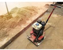
compact the freshly excavated subgrade material and sand/gravel leveling pad (if required). Add leveling pad base material in 2" layers, spraying with water to keep moist while compacting. Repeat process until final thickness of base is reached. (4" (101.6mm))
