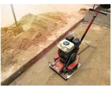
Use a vibratory plate compactor or hand tamper to compact the new excavated area. Add approximately 2" of paver base material, spraying with water to keep moist while compacting. Repeat this process until desired thickness of base is reached. (typically approx. 6") Keep in mind that any eleva on inconsistencies on the compacted base will be evident on finished paver surface.
