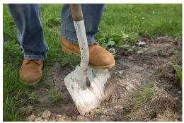
Refer to www.call811.com before digging or excavation begins. Dig entire area where pavers are planned approximately 6" deep and 6" longer and wider than desired final dimensions. Remove any grass, sod, roots, large rocks and/or organic material.
