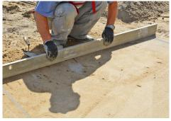
Place two pieces of 1" outside diameter pvc or steel pipe on compacted aggregate base with a comfortable workable space between the two pipes.
