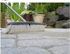
Sweep dry polymeric sand into joints between pavers after initial compaction, being sure to follow manufacturer's recommended installation instructions. You are now ready to enjoy your 4x8 Holland Paver project
