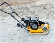
Run vibratory plate or use hand tamper to compress pavers into loose sand setting bed. Care should be taken in this step not to scuff or excessively scratch paver surface. Use of cardboard sheets or rubber mats under tamper plate are suggested.
