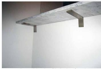
you can caulk around the edge of the brackets if you choose. This will give greater adherence to the countertop and cover any gap between the brackets and counter.
