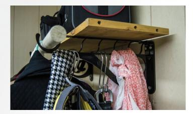
Once all the brackets are in place, you are ready to install your shelf for additional storage. Be sure you have measured to make sure your selected shelf will fit. Fasten the shelf to the brackets using the provided holes and wipe the brackets down to get rid of any handprints or other debris. Now you are ready hang your clothes, bikes, tools, plants, or signs and store your stuff on top.
