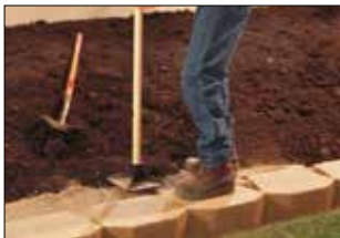
2. Place & Compact Backfill
