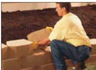
3. Install Additional Courses
