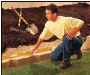
1. Prepare Wall Location
