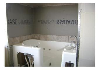
The pictures below depict the correct and incorrect alignment of the tile flange and cement board. The picture labeled incorrect shows that the cement board is not lined up properly with the integral tile flange, leaving an air gap. The picture labeled correct indicates that the cement board has been properly installed ensuring a perfect tile angle.
