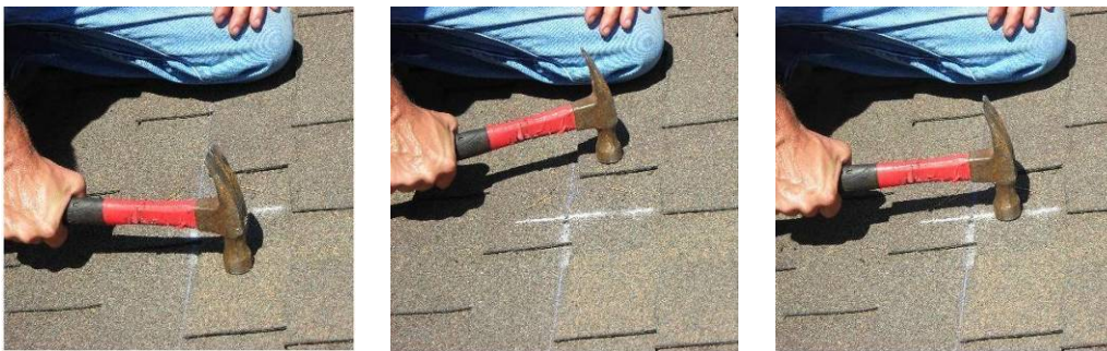
Figure 14 - Tapping across assumed rafter location to find firmest point
