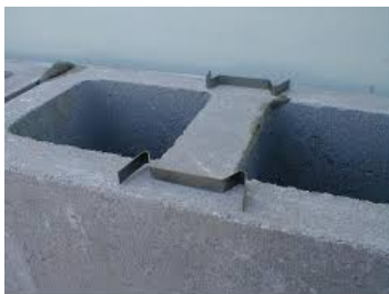
Concrete Block and Brick Spacers
