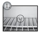
Hammer in 3 of the included Wire Clamps at the rear of your pre-existing wire shelving unit (should you have wood shelves these are not necessary just discard wire clamps) about 4 to 6 inches apart. This is for reinforcement and additional support for wire shelves.
