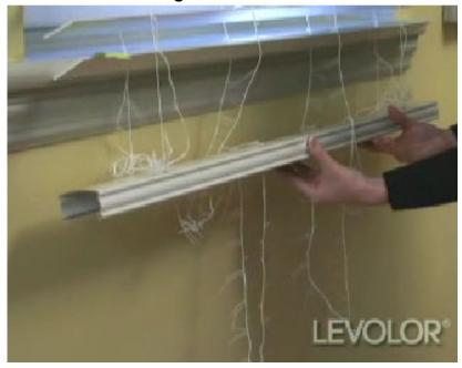
Step 7: From the open bottom side of the bottom rail pull each of the ladder cords downward as far as they will go
