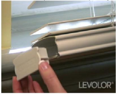
Slide out the slat in the bottom rail, exposing the inside of the rail
