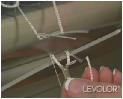
Step 8: Double check the desired length of the blind before any further cutting; then, trim all ladder cords 4 in. below the bottom rail
