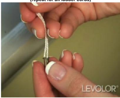
Step 10: Slide the eyelets as far inside the bottom rail as possible and crimp tightly with the pliers (repeat for all ladder cords); trim excess ladder cord 2 in. below the eyelets
