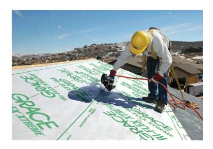
**Durability**—Unlike conventional roofing felt that typically buckles and "telegraphs" after exposure, Tri-Flex Xtreme *can withstand extreme weather conditions* and still remains flat. This is even more important when drying in the roof. It does not dry out or rot at high temperatures; it does not crack or become brittle at low temperatures; it does not shrink after hot and cold temperature cycles. Product can be left exposed for up to 120 days.
