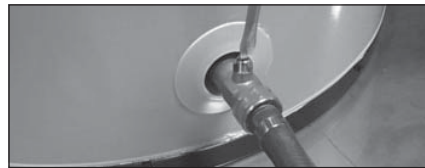
Figure 40 - Drain Valve
