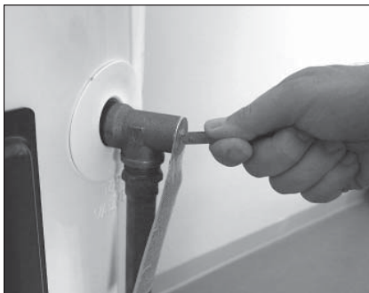
Figure 43 - T&P Relief Valve
