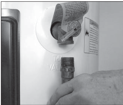
Figure 11 - Removing the T&P Relief Valve discharge pipe.
