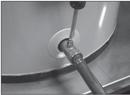
Figure 10 - Draining the old water heater.
