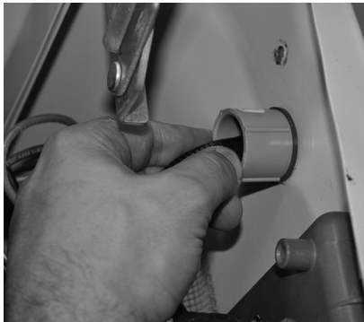
Figure 3.7 - Installing Fitting with Harness
