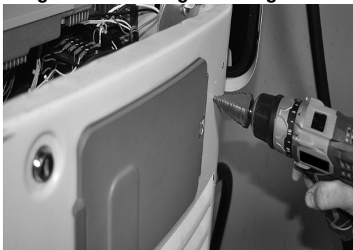
Figure 3.5 - Drilling Mounting Hole.
