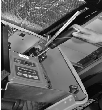
Figure 3.13 - Removing Controller Fasteners.
