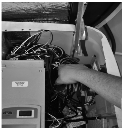
Figure 3.4 - Checking Wire Clearance
