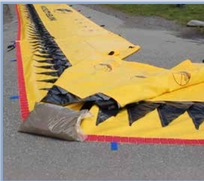
Corners created by folding material, leaving middle section on top
