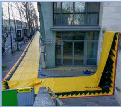
Lifting & securing the ends, helps seal the edge against water infiltration
