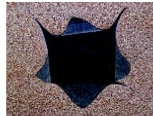
1. Cut an "X" in roofing material where blister is located. Peel back the flaps exposing the underlying surface. Allow area to dry.
