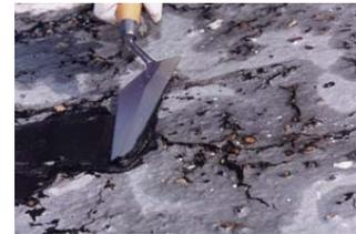
2. Cut and place a strip of **Universal Patching Fabric** into the cement. Spread more roof cement over entire repair area and let cure.
