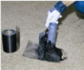
1. Apply roof cement at base of projection. Spread the cement around the repair.
