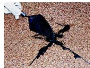
2. Trowel **Black Jack roof cement** into exposed area making sure to cover entire area. Push flaps back down to cover the underlying surface. Cover with additional roof cement.
