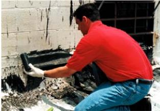
1. Flashings pulling away from walls should be reset in roof cement.
