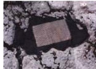
1. Cover cracked and damaged area with **Leak Stopper** or **Black Jack All-Weather Roof Cement**.
