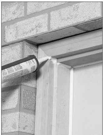
Figures 30 and 31: Caulk the jambs and the exterior trim.
