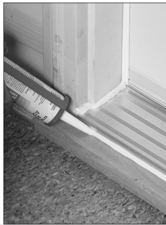
Figures 28 and 29: Caulk the sill crown and the front of the sill.
