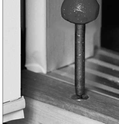
Figure 32: Raise or lower the sill by adjusting the sill screws. Some sills may have covers over the adjusting screws. These covers must be removed prior to making any adjustments.
