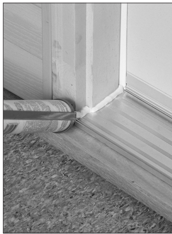
Figures 28 and 29: Caulk the sill crown and the front of the sill.
