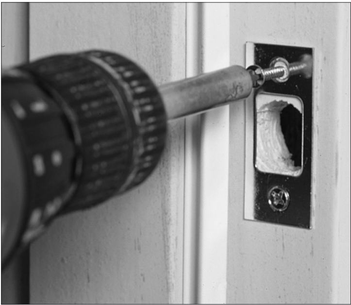
Figure 26: Screws fasten the latch plate to the door slab.
