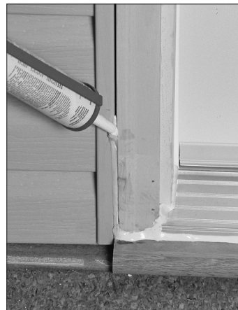
Figures 30 and 31: Caulk the jambs and the exterior trim.
