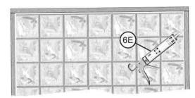
F. If your glass block panel will function as a shower wall, after about a week, coat the mortar joints on both sides of the panel with tile grout sealer for mold and mildew protection.
